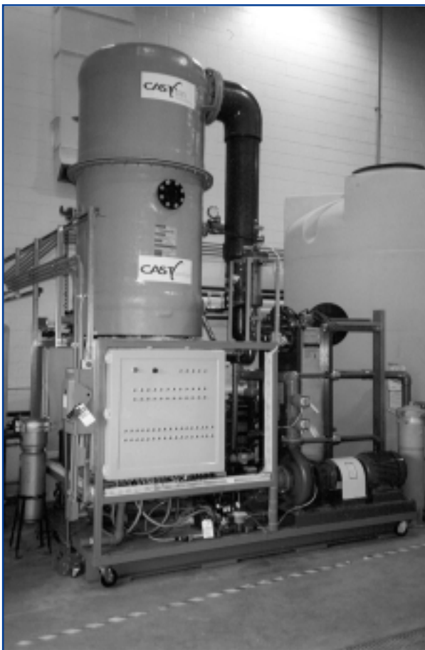
CASTion Corporation's Controlled Atmospheric Separation (CAST®) technology.
