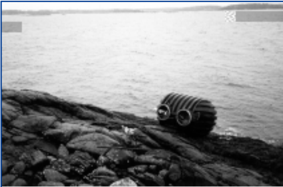
SeptiTech's tank being winched up a cliff on Fox Island, off the coast of Maine.
